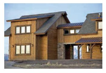
\*T&G MILLED TO NET 11/16" WITH REVERSIBLE RESAWN OR SURFACED SIDES.
